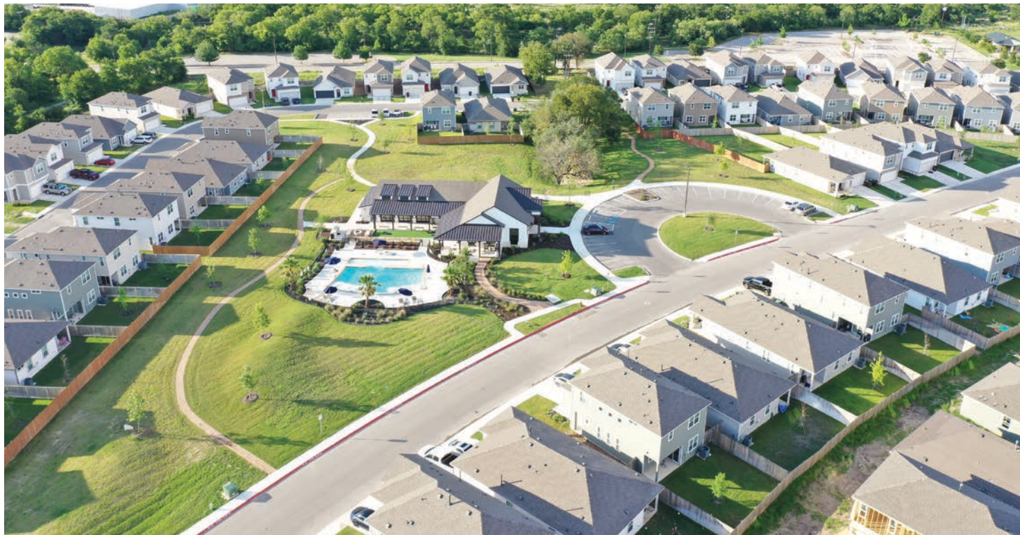
PHOTO: COURTESY AHV COMMUNITIES
