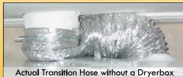
Actual Transition Hose without a Dryerbox
