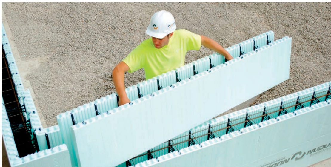
NUDURA ICFs complete the building envelope in one building step.
