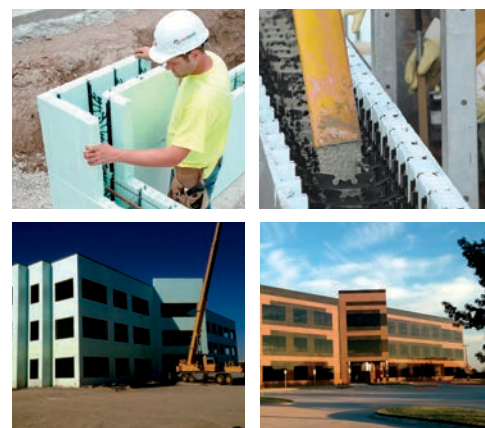
NUDURA ICFs complete the building envelope in one building step.
